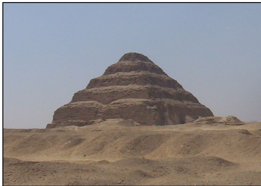
Figure 1. The stepped pyramid of Djoser at Saqqara. (Photo by A. Habermehl, 2008)
